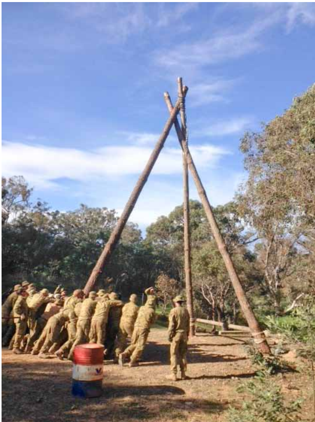
Above: 5CE Sqn members erect an aerial ropeway as part of Ex Slaters Knoll.
