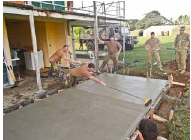
Above: 5ER Sappers Elliott and Halse finishing a concrete slab at Moem Barracks, Wewak, PNG as part of Ex Puk Puk 2014. This slab was to become the foundation for the adjoining barracks new water tanks, pumps and shower facilities. Evidently the broom handle left something to be desired in terms of length.
