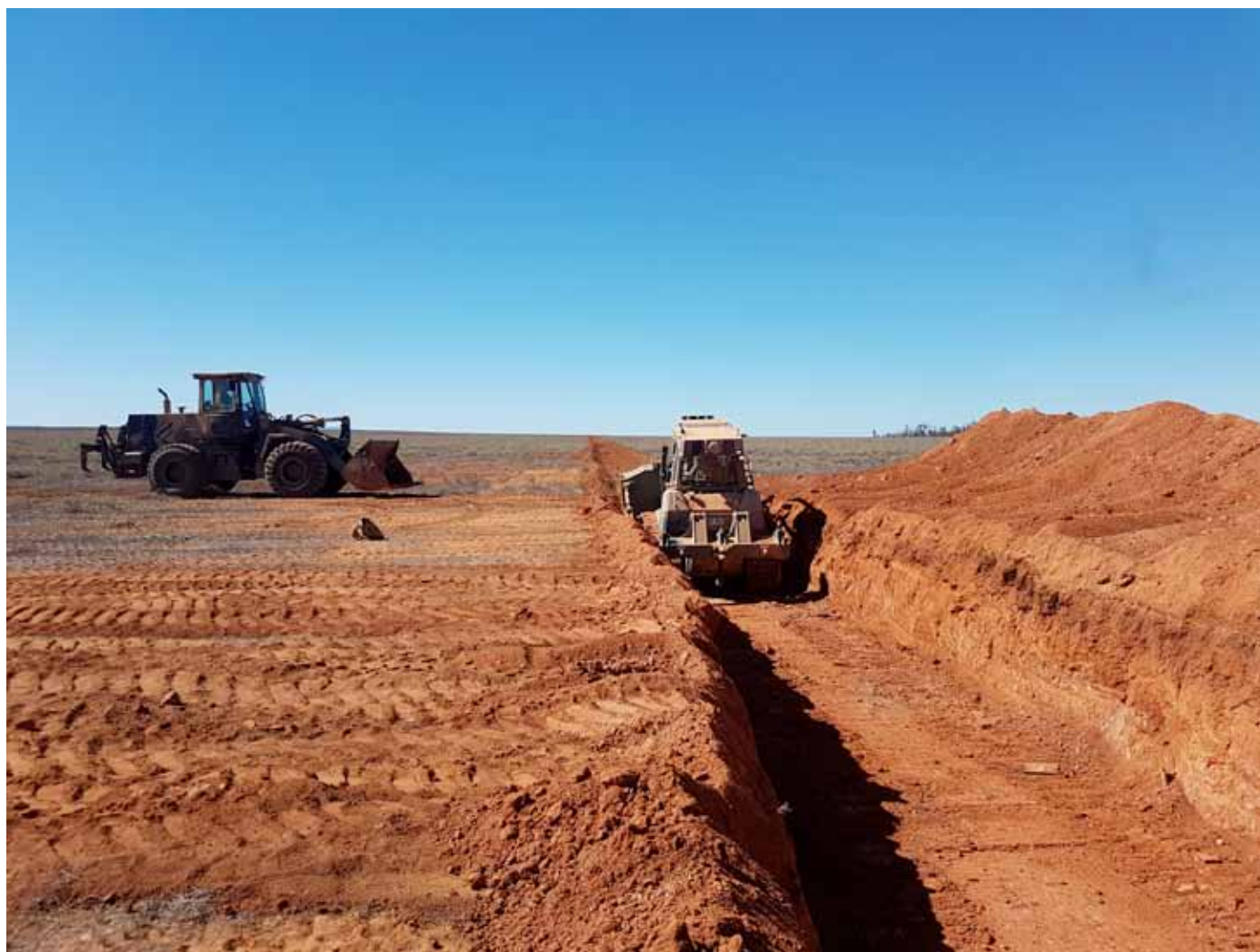
Plant Tp starts a 1.4Km tank ditch during Ex PREDATORS RUN
