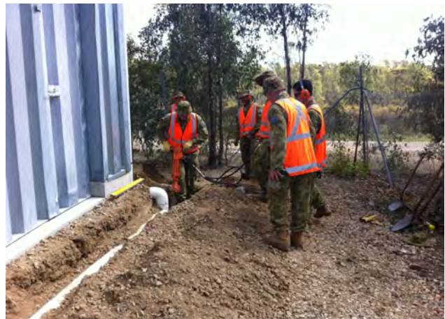
CEs from 22 using the Stanley Power Pack on the rainwater drainage system at the Lysaght Building
