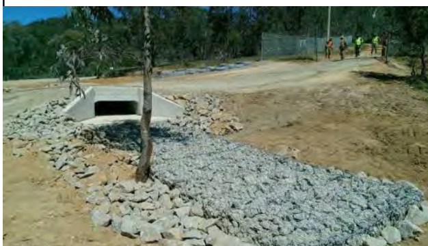
Rear access ramp remediation (culvert with wing wall and drainage) complete.
