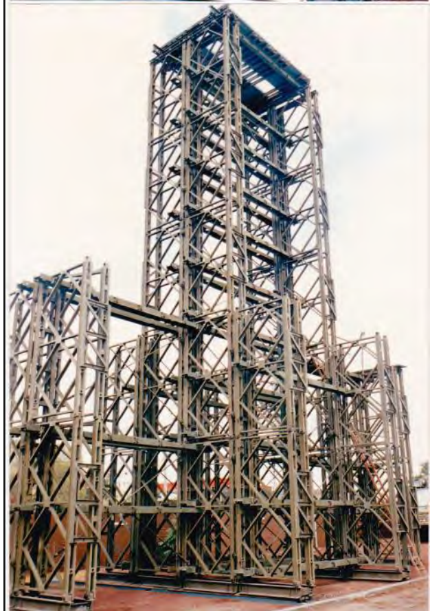
50' Bailey Tower built by 10 Fd Sqn at the Royal Melbourne Show 1989
