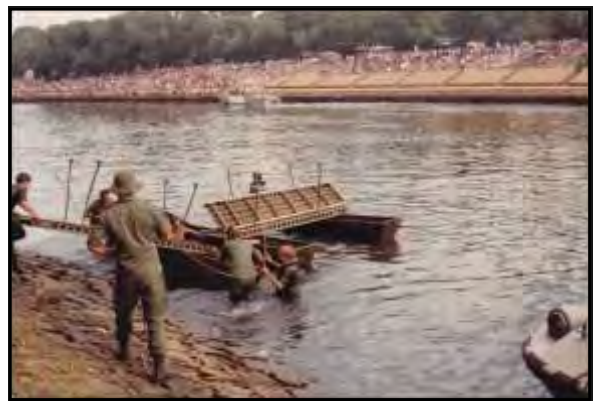
7FER engineers build a floating bridge across the Yarra River in Melbourne 1981.
