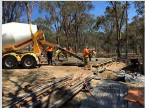
Construction Section laying foundation slab for a training shed during Ex PLATYPUS CONSTRUCTS
