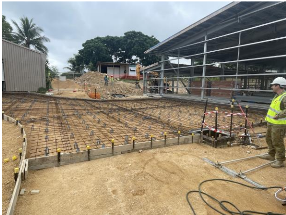
CAPT Oscar Dyer inspects reinforcing in concrete pavements at Cook Barracks.
