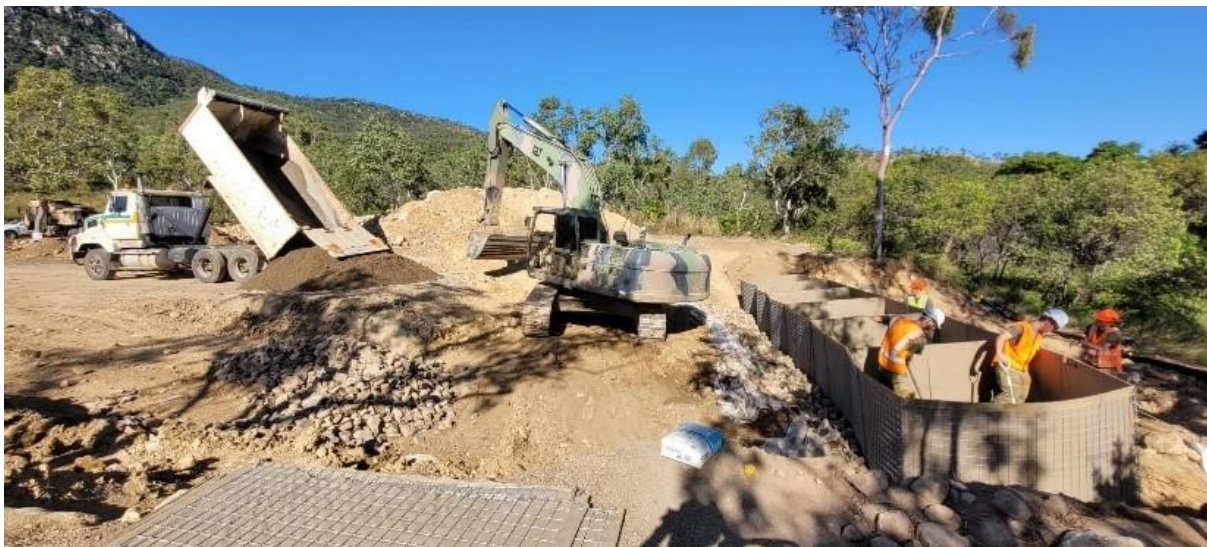
Construction Troop establishing bridge abutments for the 3 CER Bridging Precinct to support MGB and DSB training.
