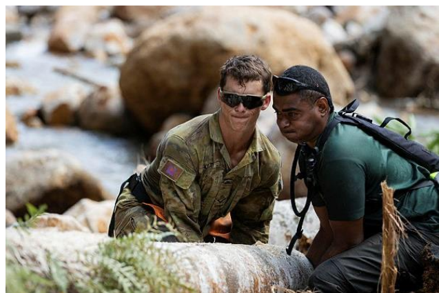
10 TP and RFMF constructing Corduroy Road in Huonbrook, NSW
