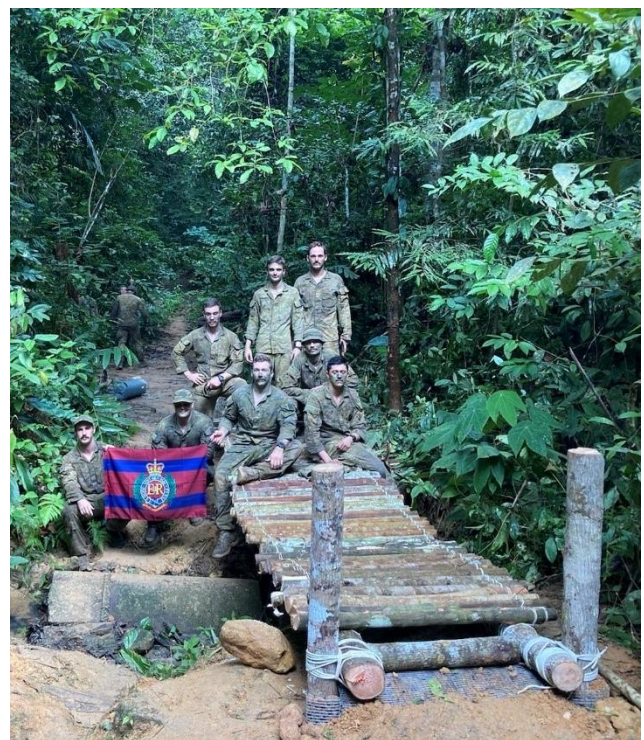
Sappers from 9 Fd Sqn construct a foot bridge
