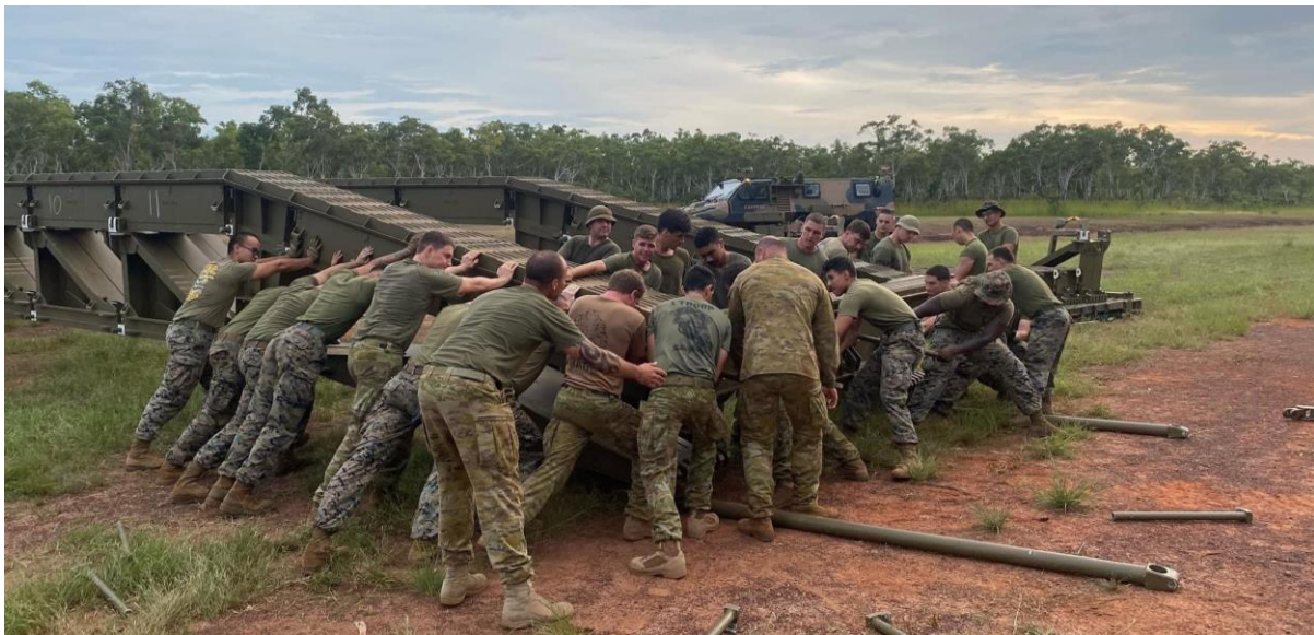
Members of 1 Troop and the Marine Rotational Force – Darwin wrestle with the bankseat beam on the Medium Girder Bridge.
