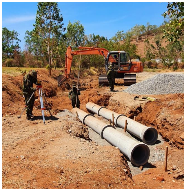
1 CER plant operator SPR Ben 'Shooter' Masterson working with JGSDF and F-FDTL to emplace a new culvert at Metinaro Military Base in preparation for the wet season.
