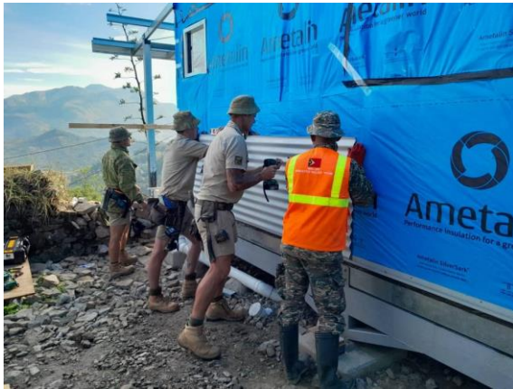
External cladding commences on the accommodation block constructed at the remote F-FDTL border outpost in Timor-Leste.
