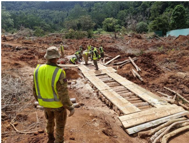
SPR Huxley and RFMF Engineer moving logs for non-equipment bridging in Huonbrook, NSW
