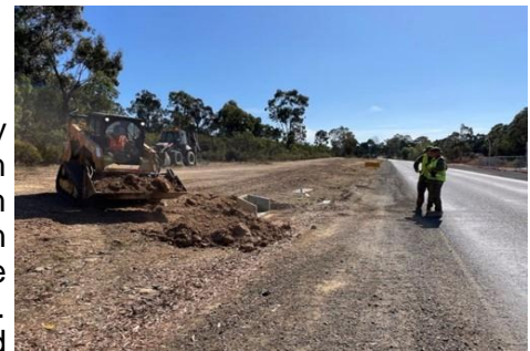
Members of 105 CONST SQN emplacing culverts to improve the longevity of the new PMA walking track
