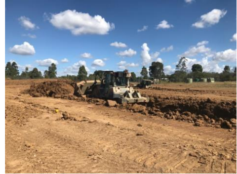
104 CS constructing M1A1 tank hides with medium dozers
