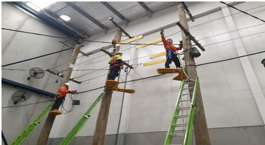
Members of the Adv Field Power Generation Course training on overhead power distribution systems.
