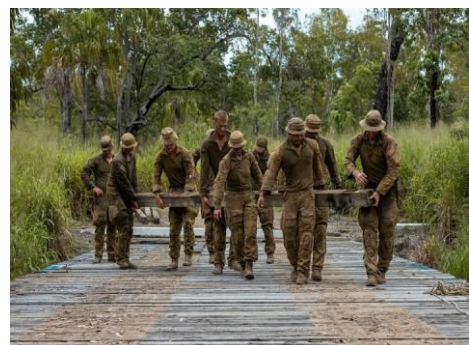
14 Troop Sappers remove timber planks from Elanora bridge in preparation for demolition
