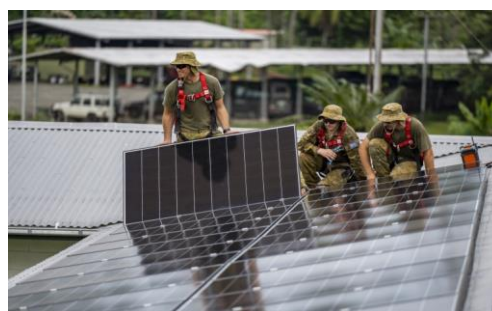
6 ESR members installing a solar system on the 2PRIR Regimental Aid Post
