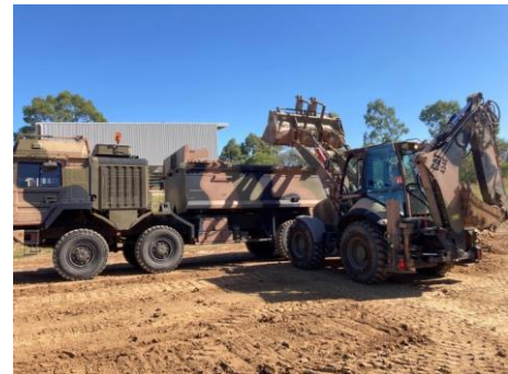
104 CS conducting earthmoving tasks using a backhoe/ HX-77 dump configuration
