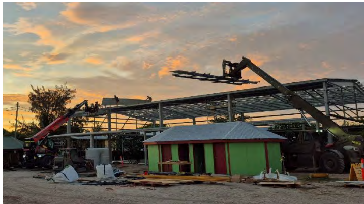
2 TP construction of the portal frame on Poruma Island.
