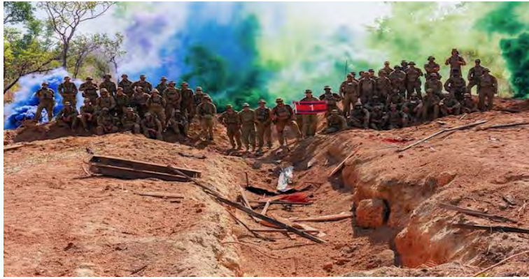
1 FD SQN with the remnants of an NEB post initiating reserve demolitions on Exercise Amphibian Walk.
