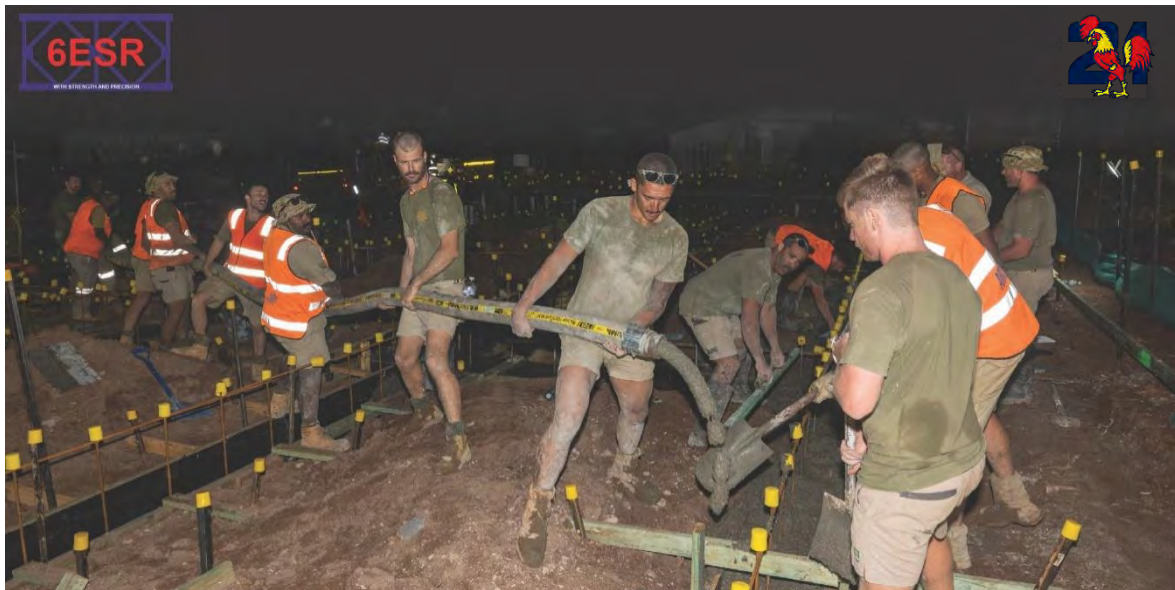
Members of 1 TP constructing the community hall on Erub Island.
