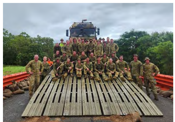
MGB constructed on the Bruce Hwy during NQLD Floods Feb 2025
