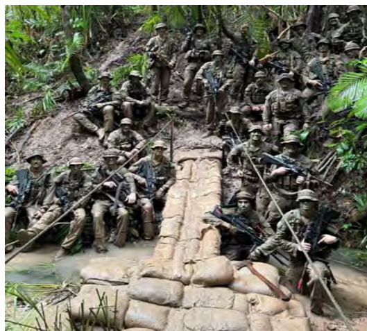
E11 with an improvised bridge they constructed whilst on the Regional Warfighter Exercise in Tully.
