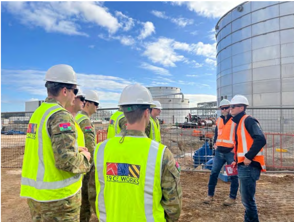
Image 11 – Upper South Creek, Advanced Water Recycling Centre 19 CE Works Site Visit.
