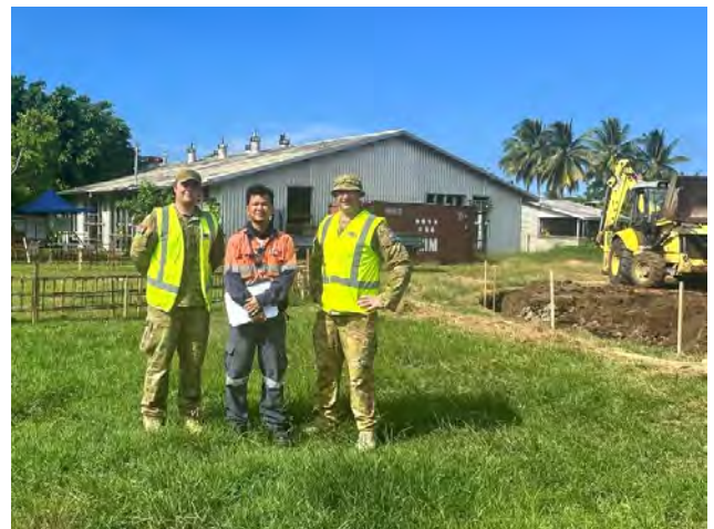
CAPT Max Cubis and CPL Andrew Ramiro with Mr Eric Carumba during the construction of the 1ML water tank at Moem Barracks
