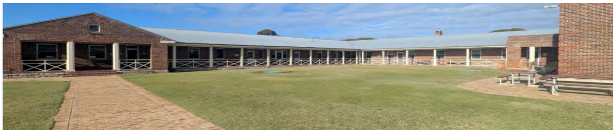
Kingston Barracks, Rottnest Island post refurbishment by members of 13 ER
