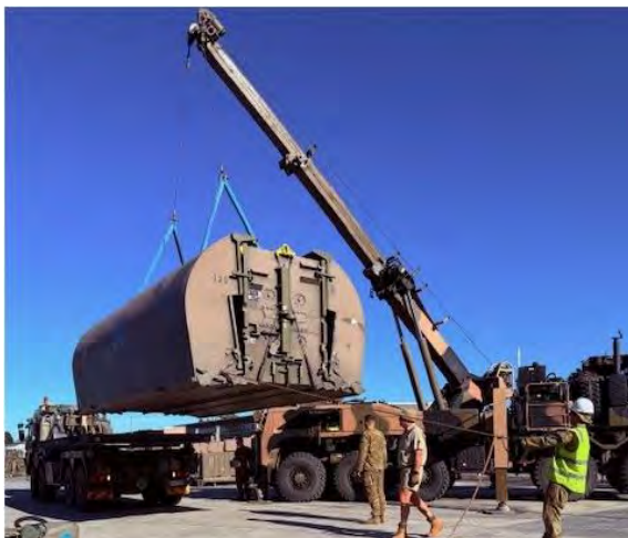
45M facilitating bridging relocation
