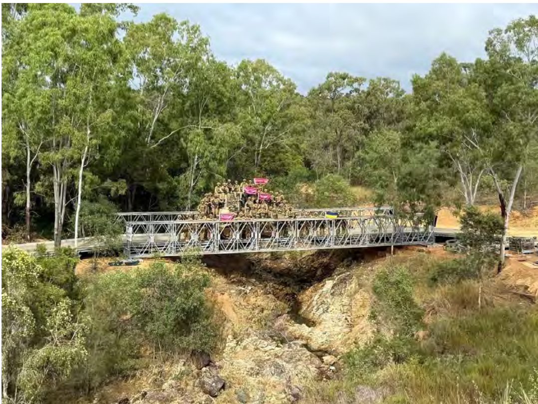
17 Construction Squadron's Fixed Modular Bridge
