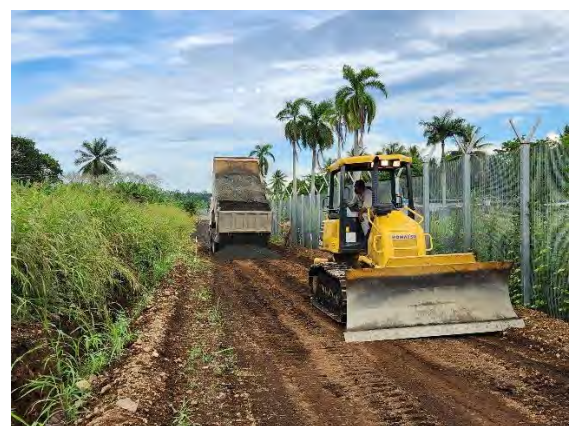
Construction of the Igam Barracks Perimeter road during Ex Puk Puk 25
