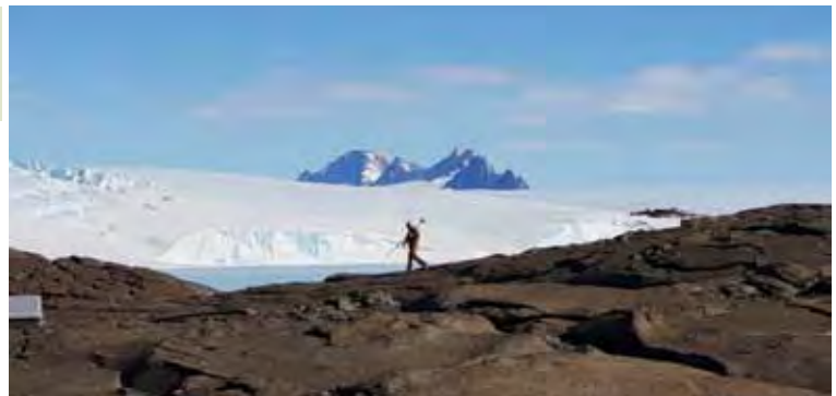
CPL Bradley Smart surveying inception phase of a new runway for Mawson Station.
