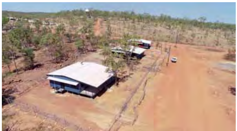
Completion handover for one of the new houses, CAPT Jonathan Glover, WO1 Richard Hicks, NIAA rep, Building Crew
