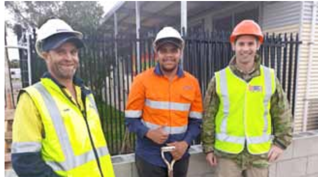
Adam Billington, site manager Ballardong Pindan, Indigenous trainee, Ruban Windlass and 19 CE Works project engineer, CAPT Tim Doust
