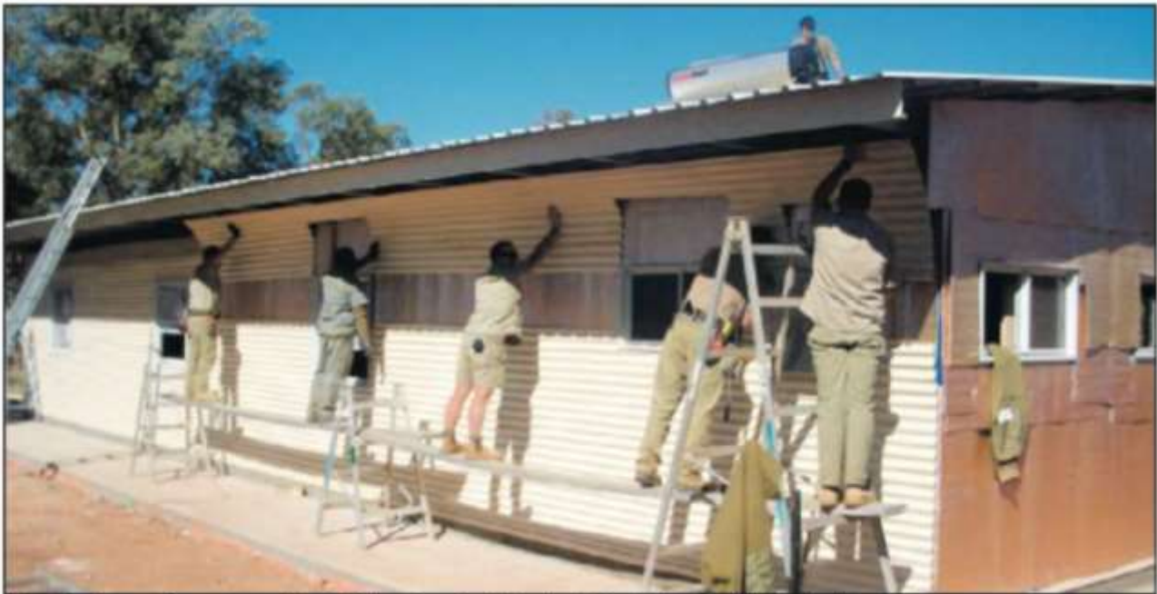
Nearly done: Sappers add cladding to a building in Pukatja in South Australia.
