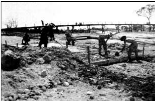
Pouring the main ramp section.
