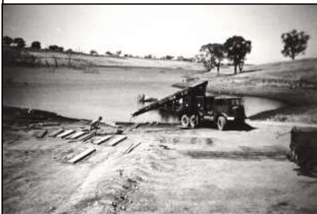
Placing the precast concrete planks.
