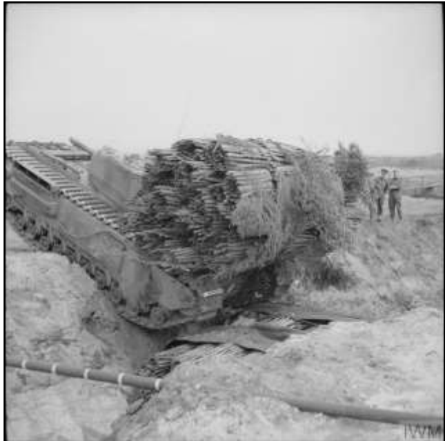
Fascine carrier adding another level to a partly filled ditch
