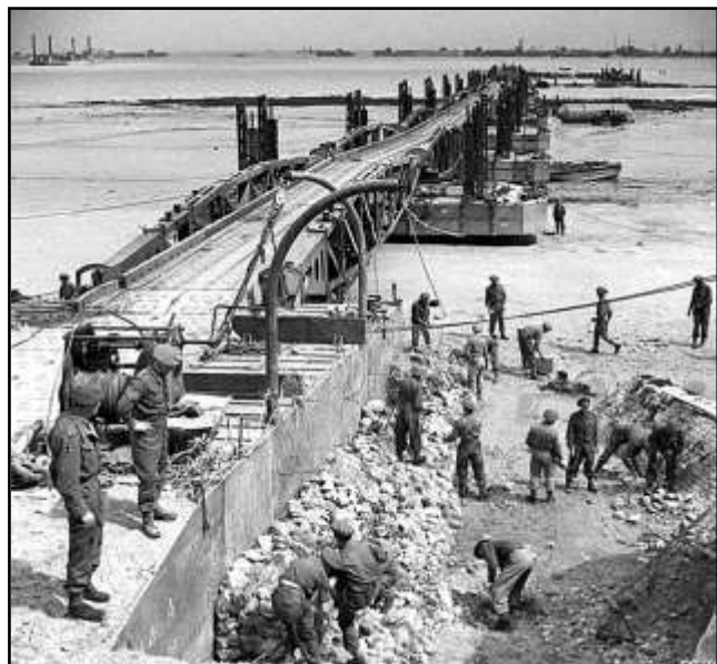
June 14, 1944, Arromanches, France. Royal Engineers working on the roadway leading to the Mulberry artificial harbour. This enabled a much more efficient unloading of all types of stores and equipment.
